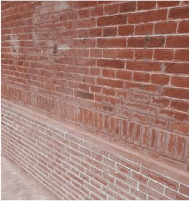
Pilot restoration of the worn-out bricks in the historic CASFOS building
