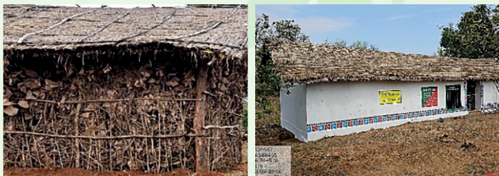
Fig. 7: Temporary Phadi House Fig. 8: Semi Permanent Phadi House
