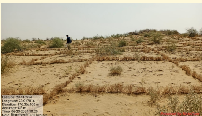
Figure 6. Checkboard fences installation on sand dunes
